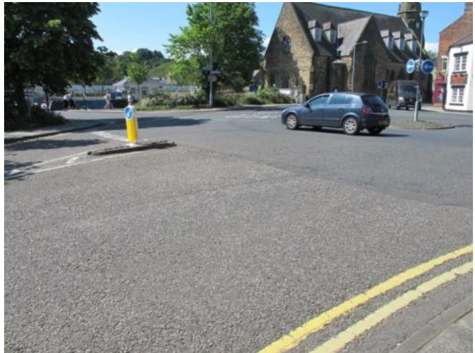
Figure 4: Damside roundabout at Gas House Ln is a difficult junction for cyclists and pedestrians to cross.
