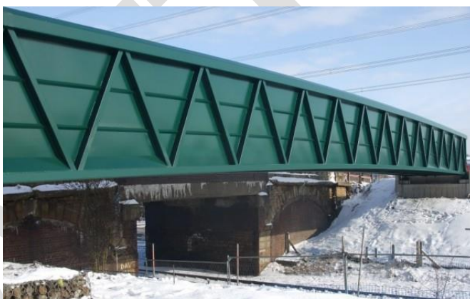
Figure 18: 32m fully clad footbridge over the railway between Halfway and Kilamarsh.
