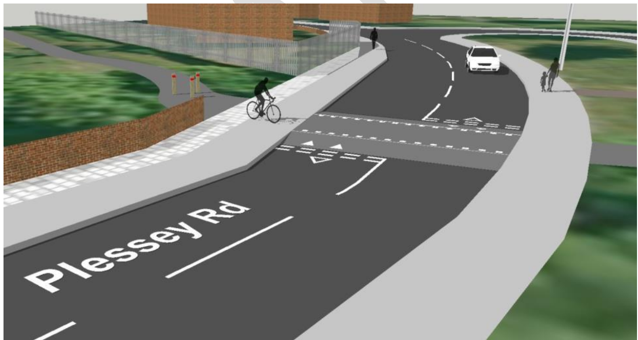
Figure 7: Raised table pedestrian and cycle priority crossing over Princess Louise Rd.
