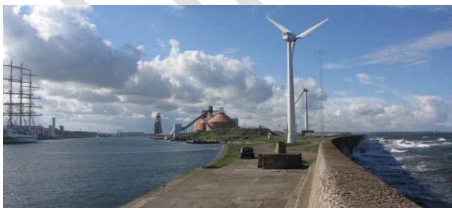
Figure 18: Coastal views from Blyth Pier
