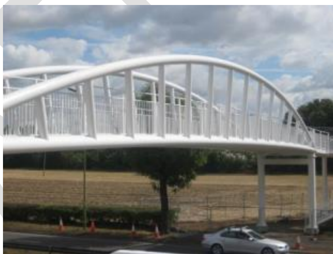
Figure 17: A prefabricated footbridge spanning a busy trunk road.
