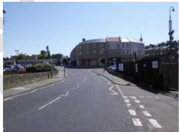
Figure 4: Dispensary St lacks suitable crossings for pedestrians.
