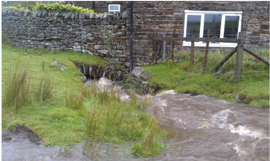
Plate 2: The entrance to the culvert in bank full conditions at Merit Hall, Burnstones
