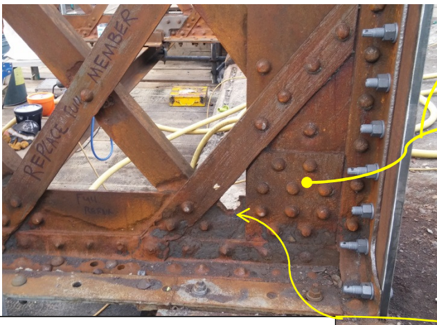
Web splice plate 1mm (1/32”) thick, originally was 10mm (3/8”) thick. In places there is total loss of section .
