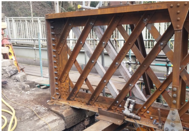
Condition of the bridge, before full repair
