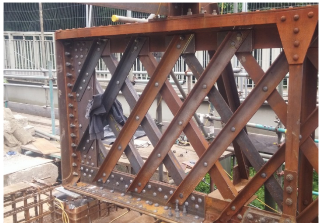
Completed full repair
