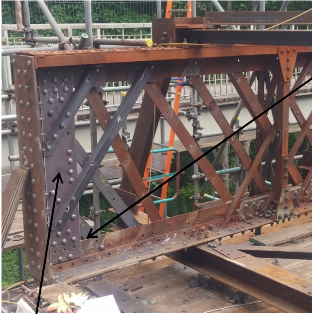
Vertical cover plate, as member had sustained significant corrosion, not the number of web members which have been removed.
