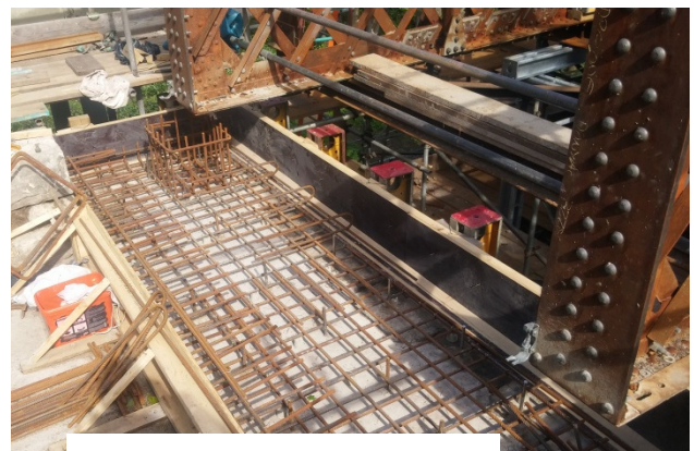
5. Bearing shelf reinforcement being installed
