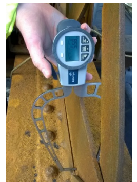
Truss being inspected and measured This determines which members are to be repaired.
