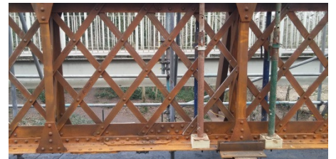
Truss after wet blasting, Wet blasting removes the lead based paint to make it safe for following trades to repair the truss
