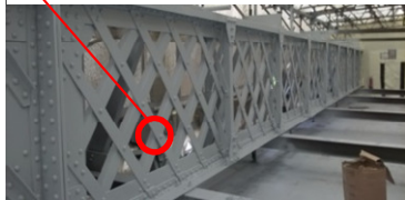
Truss after first under coat note the matt appearance
