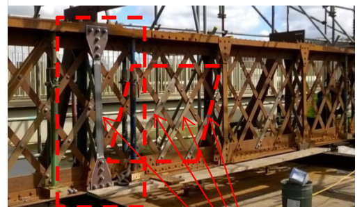
Truss sympathetically repaired The bridge is not listed, however in order to maintain its appearance the truss is repaired in keeping with its original appearance.
