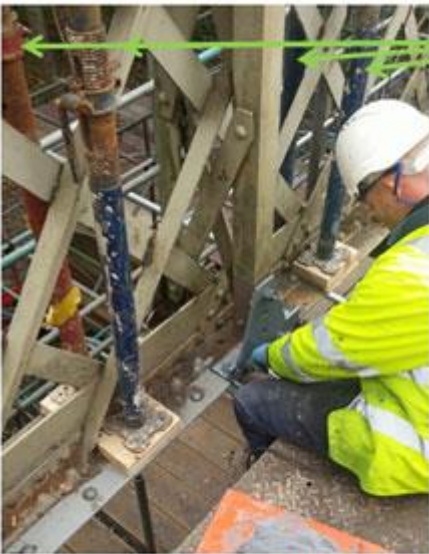
14 October – Gusset plate and angle fixed to bridge. Belzona repair metal used to provide a good contact between all elements.
