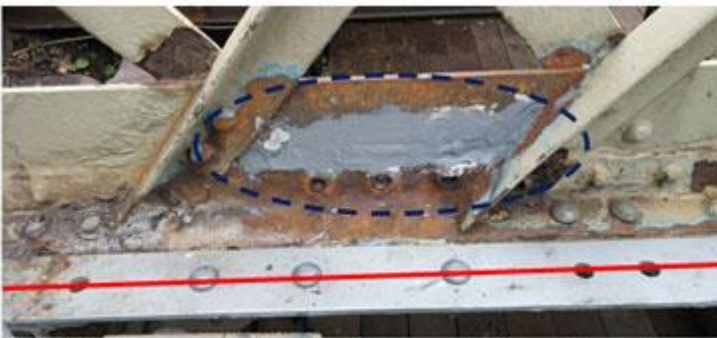
25 Sept 2014 – repair after installing Belzona, note 10mm thk overplate to bottom chord is now installed
