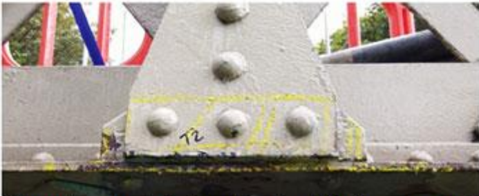
29 August - yellow chalk shows the extent of surface prep required at the U-frame stiffeners
