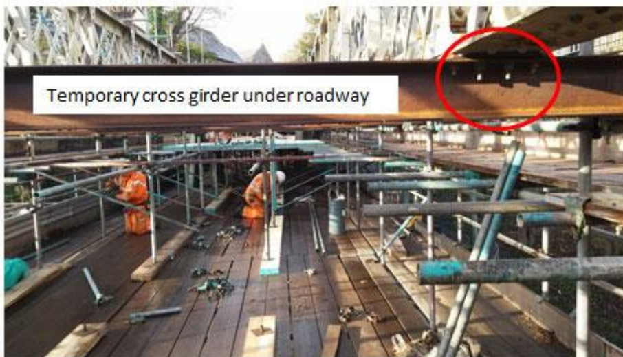
Photograph taken 12 November 2014 Scaffold beneath the road is being constructed. For connection detail (within red circle) see photograph below.
