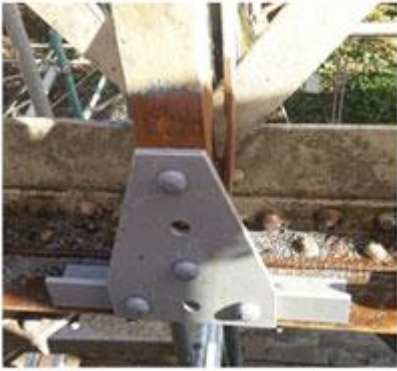
10 October – existing gusset plate and angle replaced with new elements. Note angle is not yet fixed to bottom chord.
