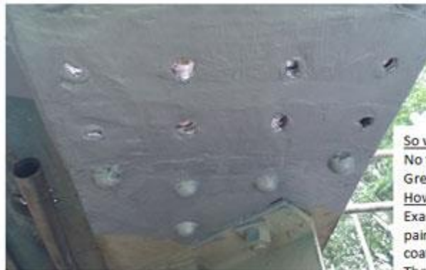
19 Sept – bottom chord soffit after repair and painting The holes are for a cross girder and have yet to be reamed out.
