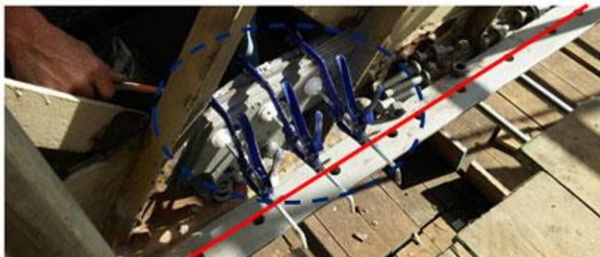
26 Sept – web plates installed (both faces), with 10mm thk overplate beneath
