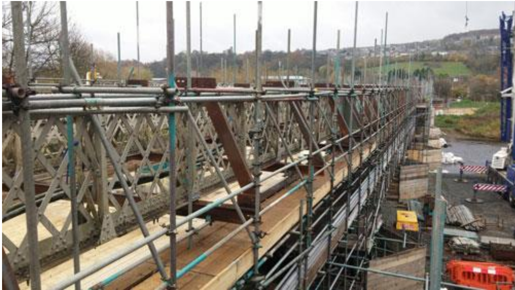
Photograph taken 12 November 2014 showing knee braces along upstream truss. Note scaffold level is now within 500mm (20") of the old road level.
