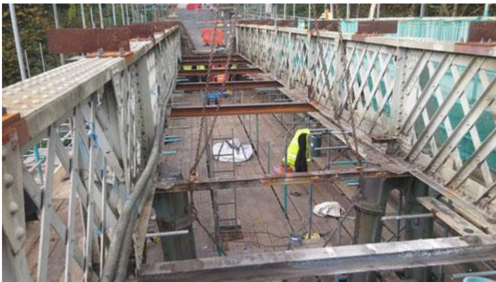
Photograph taken 27 October 2014. The roadway to span 1 (nearest Ovingham) has been removed showing temporary bracing (five furthest away) and existing cross girders (two nearest).
