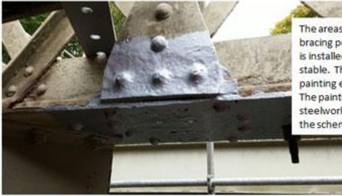
17 Sept – gusset plate and bottom chord soffit painted
