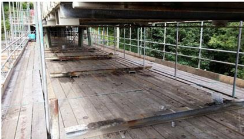
Photograph taken 22 August 2014 looking towards Ovingham Cross girders removed from span 2
