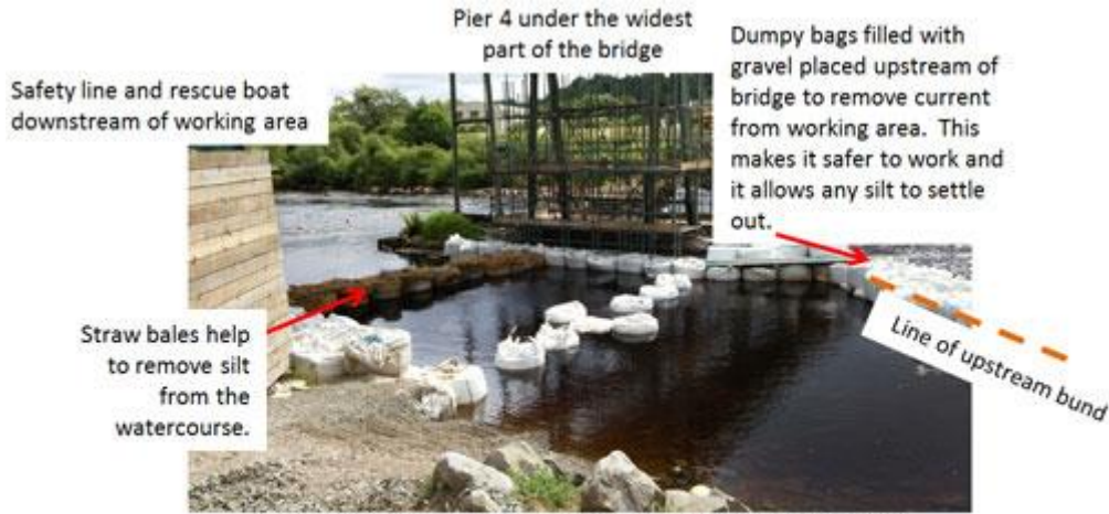
Photograph taken 30 July showing temporary works in the river, in order to build scaffold supports around bridge legs. River levels were low, typically around 0.4m, as measured at Bywell gauging station. River levels are available from the Environment Agency's website.
