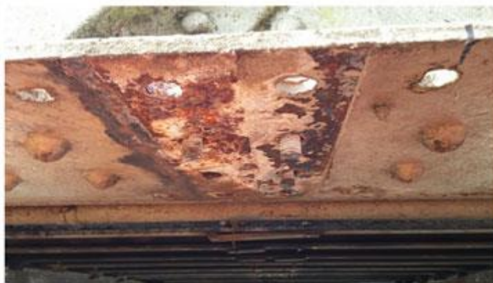
Photograph taken 22 August showing typical condition of bottom chord soffit, where cross girder was fixed to truss
