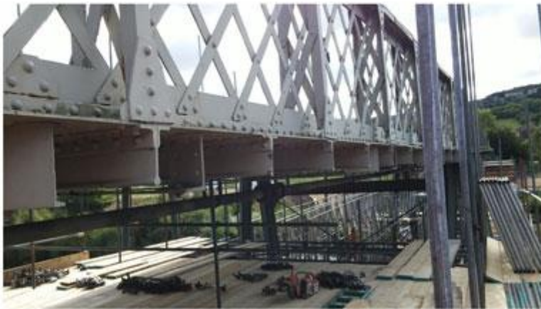
Photograph taken 22 August, inspection of the scaffold foundations demonstrated they were undamaged.
