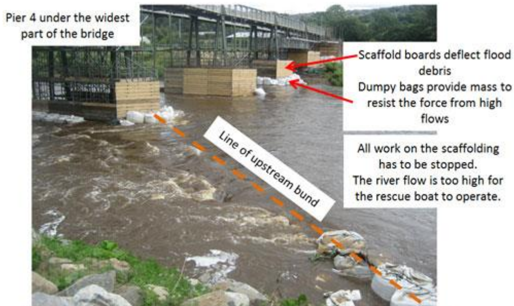
Photograph taken 11 August showing the river level covering the upstream bund
