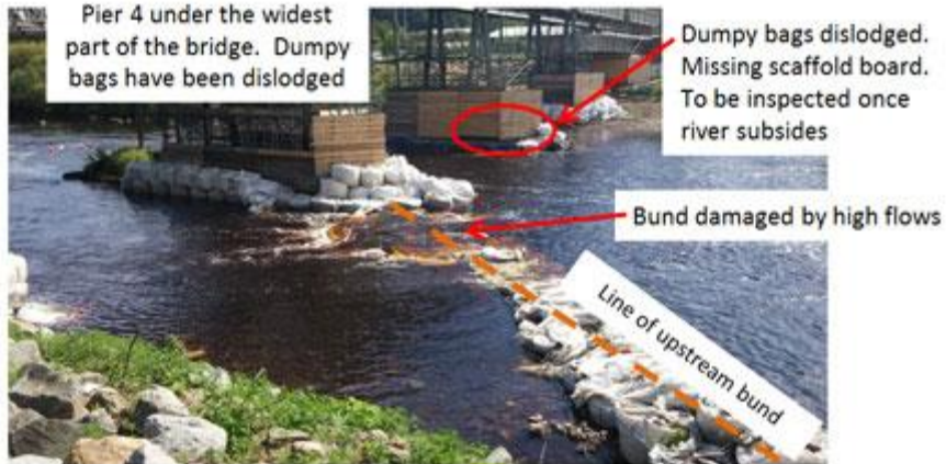
Photograph taken 18 August the river level has dropped, but not enough to assess the damage from heavy rainfall over the weekend 9/10 August
