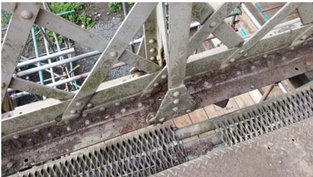
Photograph taken prior to grit blasting
