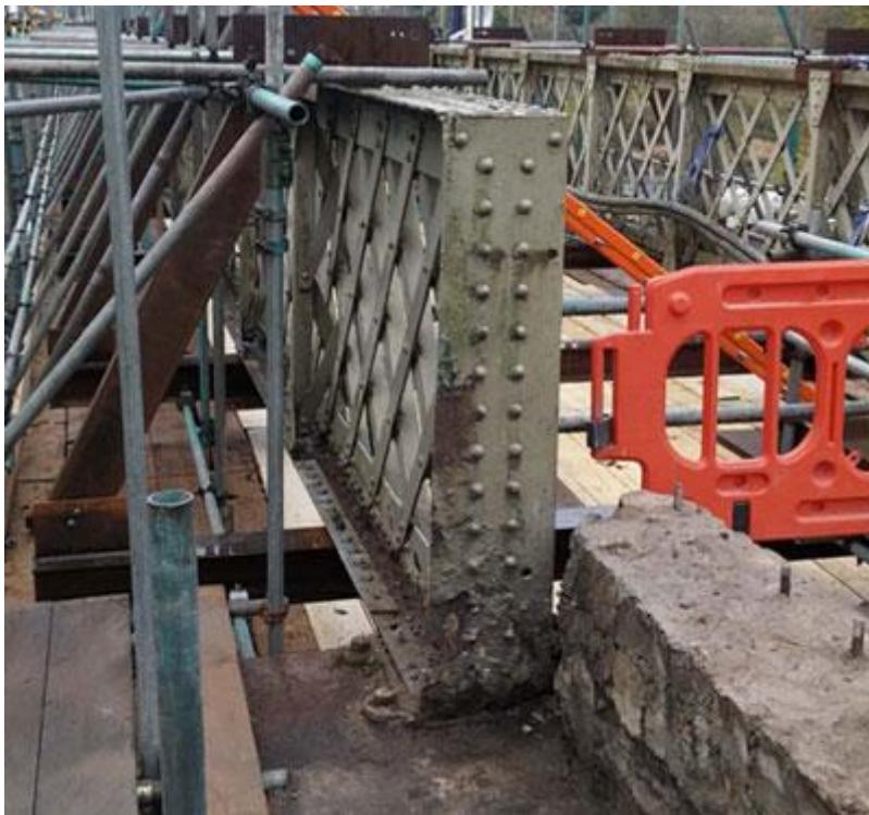
Photograph taken 12 November 2014, Showing corroded end stiffener in place
