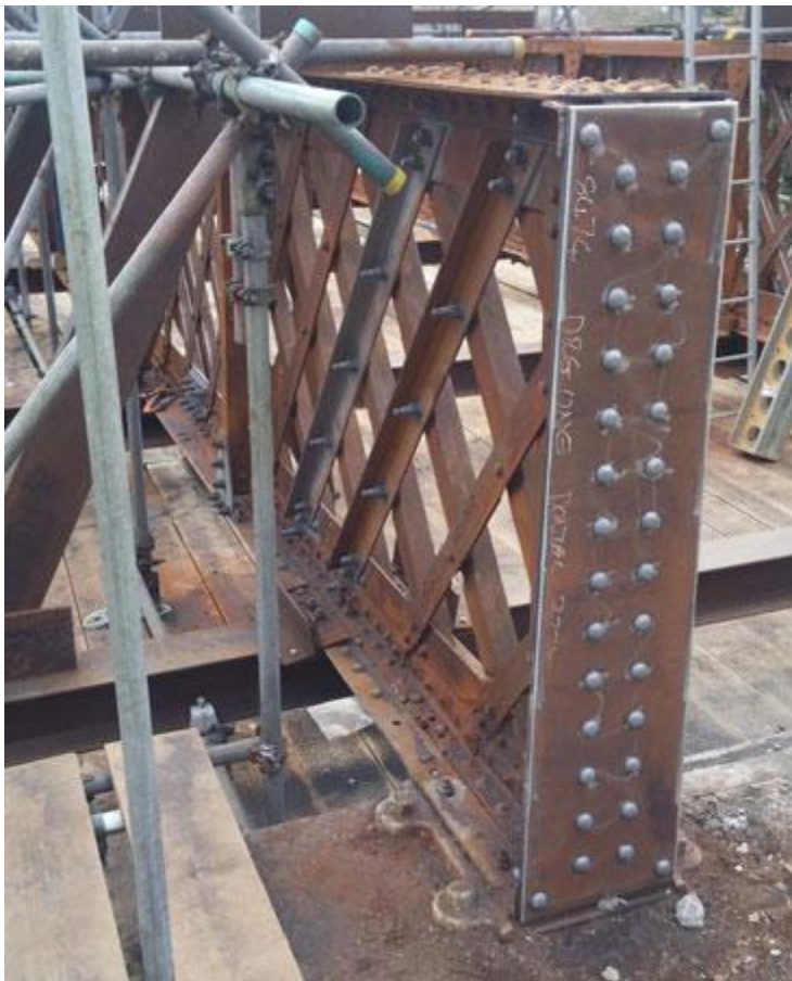
Downstream Truss, Bay one, End Stiffner
