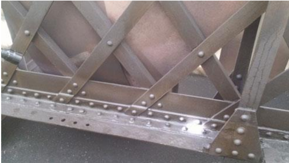
Photograph taken 18 December 2014, after test blast
