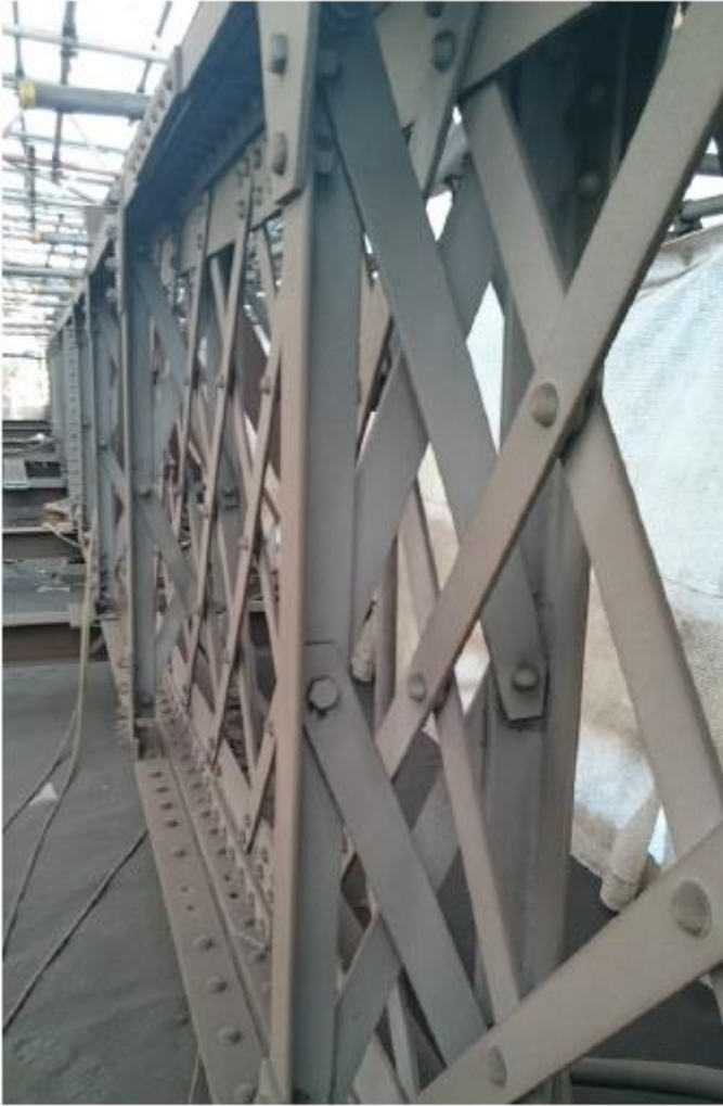
Photo taken 28 April General view along truss showing blasted truss
