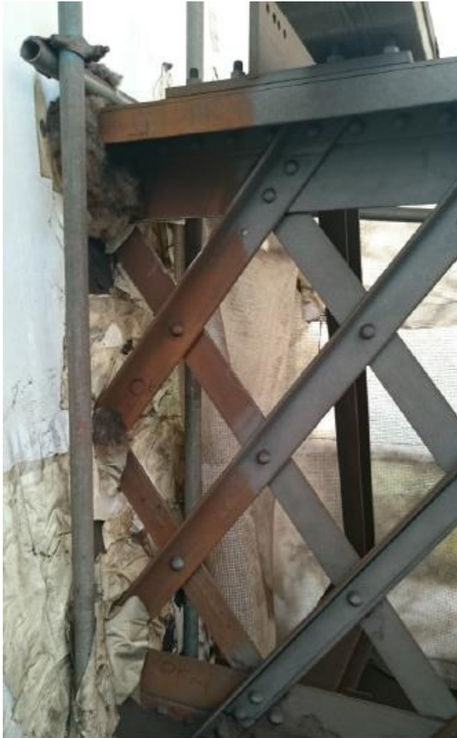
Photo taken 28 April Grit blasted truss next to rusted truss.
