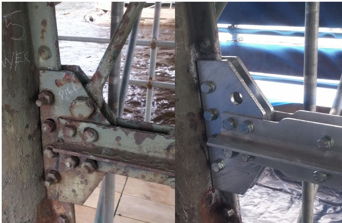
Existing & New Horizontal Cross Bracing
