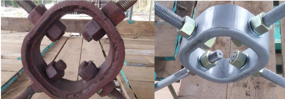
Existing & New Diagonal Tie Bracing
