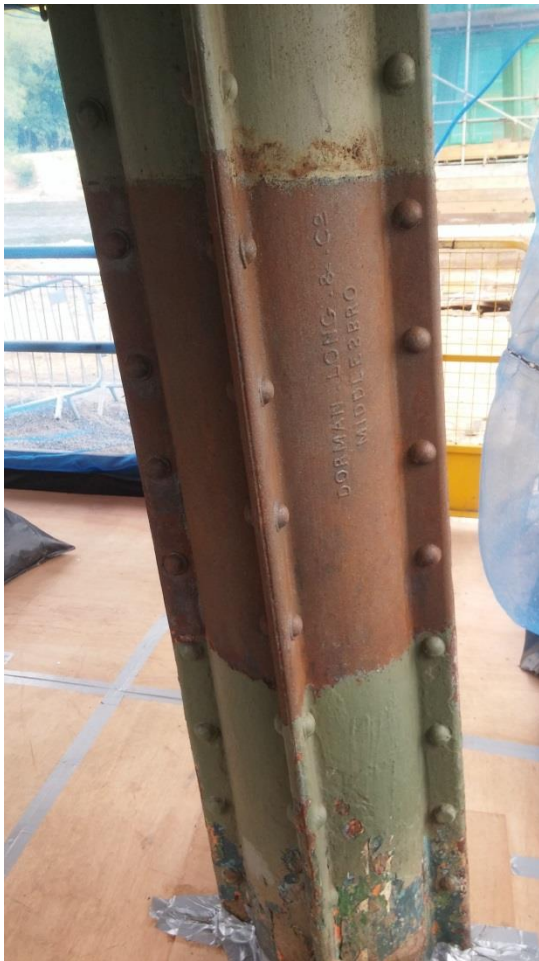
Trial of mechanical surface preparation for the application of the new paint system. picture on the left shows the surface after the existing lead based paint has been removed, the picture of the right shows the required standard for painting.
