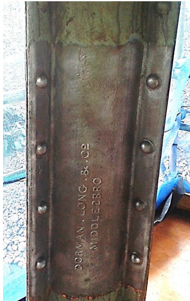
Trial of mechanical surface preparation for the application of the new paint system. picture on the left shows the surface after the existing lead based paint has been removed, the picture of the right shows the required standard for painting.
