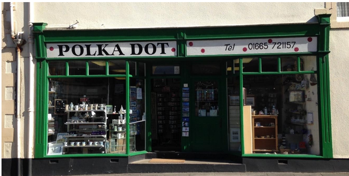
Example of traditional shop front in Seahouses
