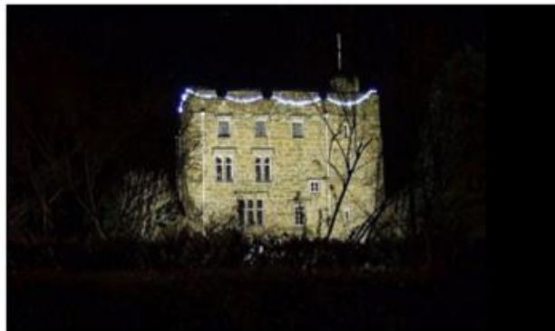
Horsley Tower, which dates from the late 15 th century
