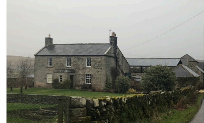
Figure 46: Traditional rectangular farmhouse with gable roof at Cockhall
