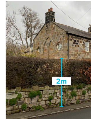
Figure 54: Terraced garden with retaining stone boundary wall and hedgerow, Eglington
