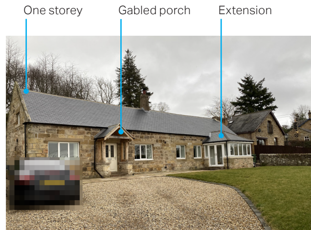
Figure 66: One storey conversion in Eglingham
