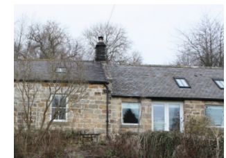
Water tabling on conversion
