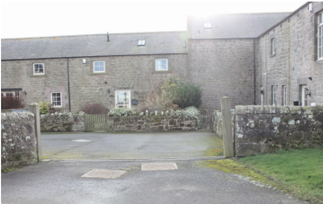
Figure 47: Farmstead conversion in North Charlton
