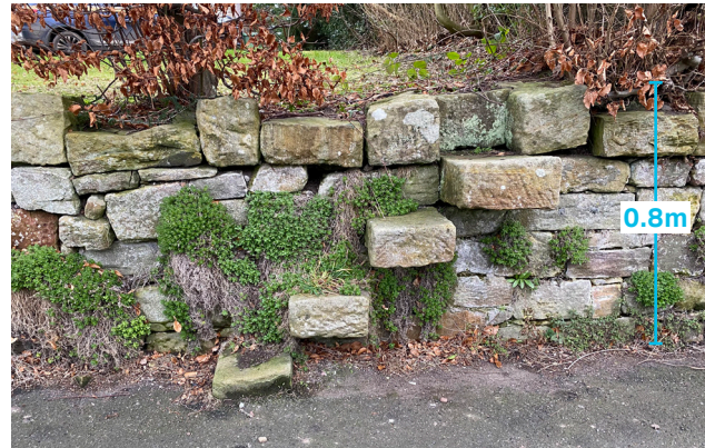
Figure 53: Mounting steps with squared crenellation coping, Eglington
