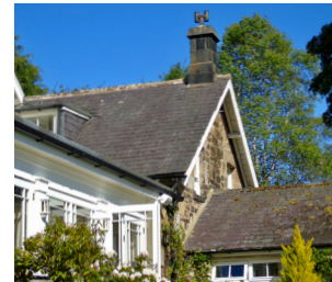
Split level roofs
