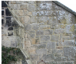
Loosely laid courses
