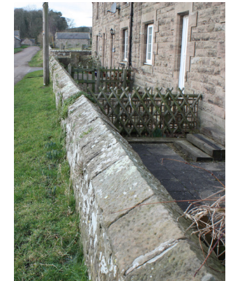
Figure 55: Saddle (pointed) coping stones, North Charlton
