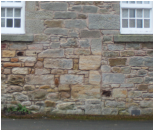
Sandstone rubble wall
