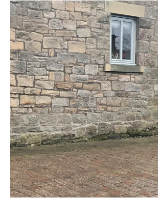
Figure 73: Natural stone (sandstone) is used as the main building material and brick used for some surfacing
