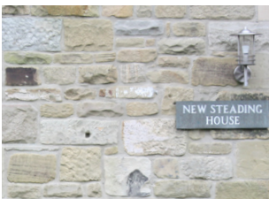
Mortar tone matches sandstone
