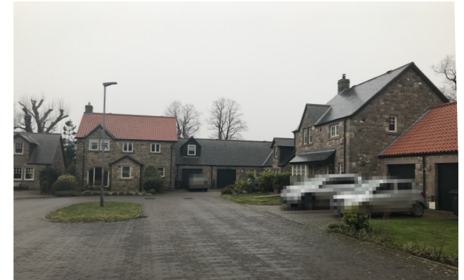
Figure 76: Roofs have been designed to vary; there is a mixture of heights, materials including red clay pantile and welsh slate, with features including the varied placement of porches, dormer windows and chimneys
