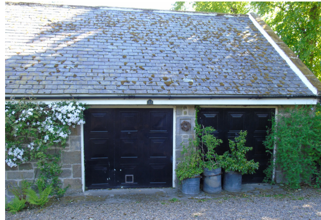
Figure 36: Garage at property in Eglington
