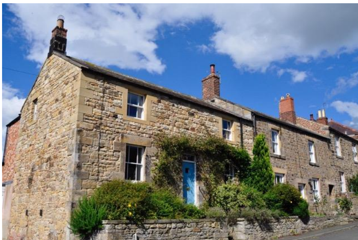
Figure 12: Traditional buildings in Acomb Conservation Area
