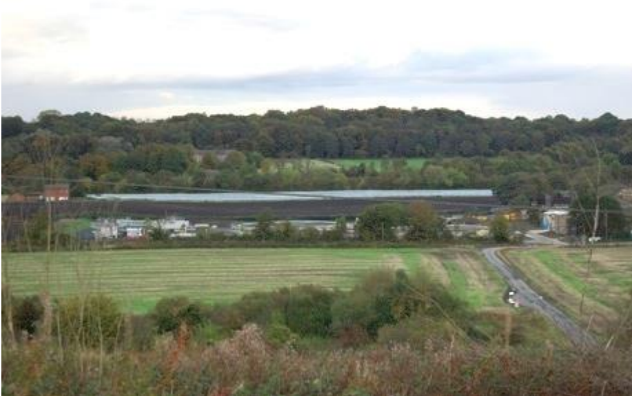
Morpeth Sewage Treatment Works
