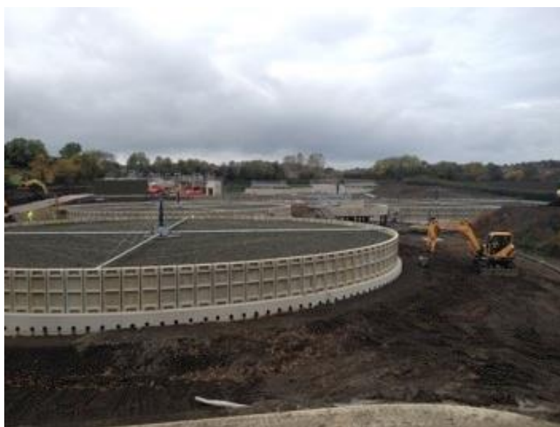
Development of Morpeth Sewage Treatment Works
