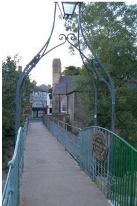
The Chantry Footbridge
