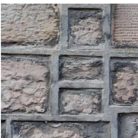
It is a misconception that hard pointing will prevent water ingress. Impermeable cement mortars actually accelerate stone decay and damp as well as have a negative visual impact. Wherever possible, mortar should be carefully matched with existing pointing.
