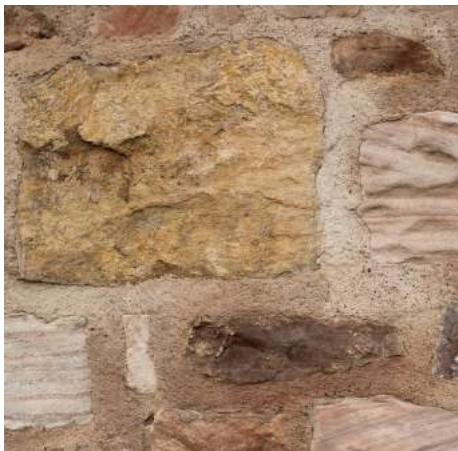
Less characterful brick (e.g. an engineering brick) tends to be intrusive when used for modern repairs, alterations and additions. The same goes for repairs and alterations which use brick or blockwork instead of stone. Poorly matched colour, size, texture and bonding of stone is equally damaging.
