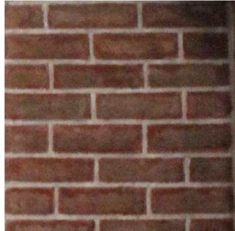
building system that is prevalent throughout the conservation areas. Lime mortar mixes should be retained and used in conjunction with traditional materials. These mortars are available in variety of shades, and sometimes crushed shell is added to give the building sparkle.
