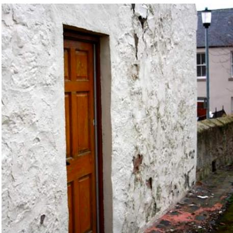
Painting sandstone detailing, particularly door and window surrounds, destroys the rich historic patina of time that characterises mature unpainted sandstone and, depending on the use of colour, can give the building an over-elaborate appearance inappropriate for the area's often understated architecture.
