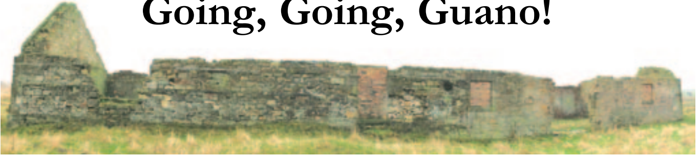
Composite view of Alnmouth's Guano Shed, north elevation.
