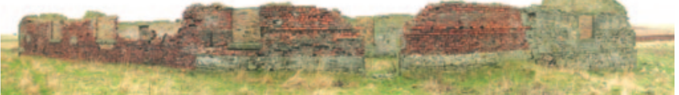
Composite view of Alnmouth's Guano Shed, south elevation.
