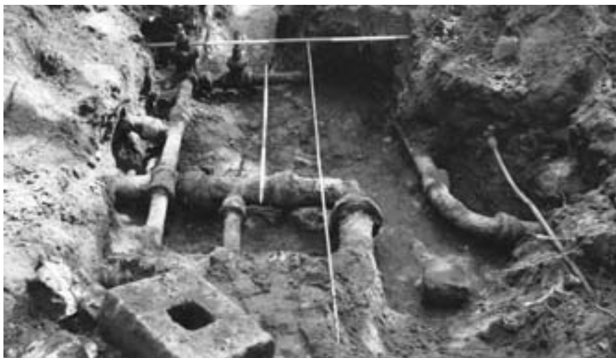
Complex of Armstrong's cast-iron pipes. Photo: Dave Reed
