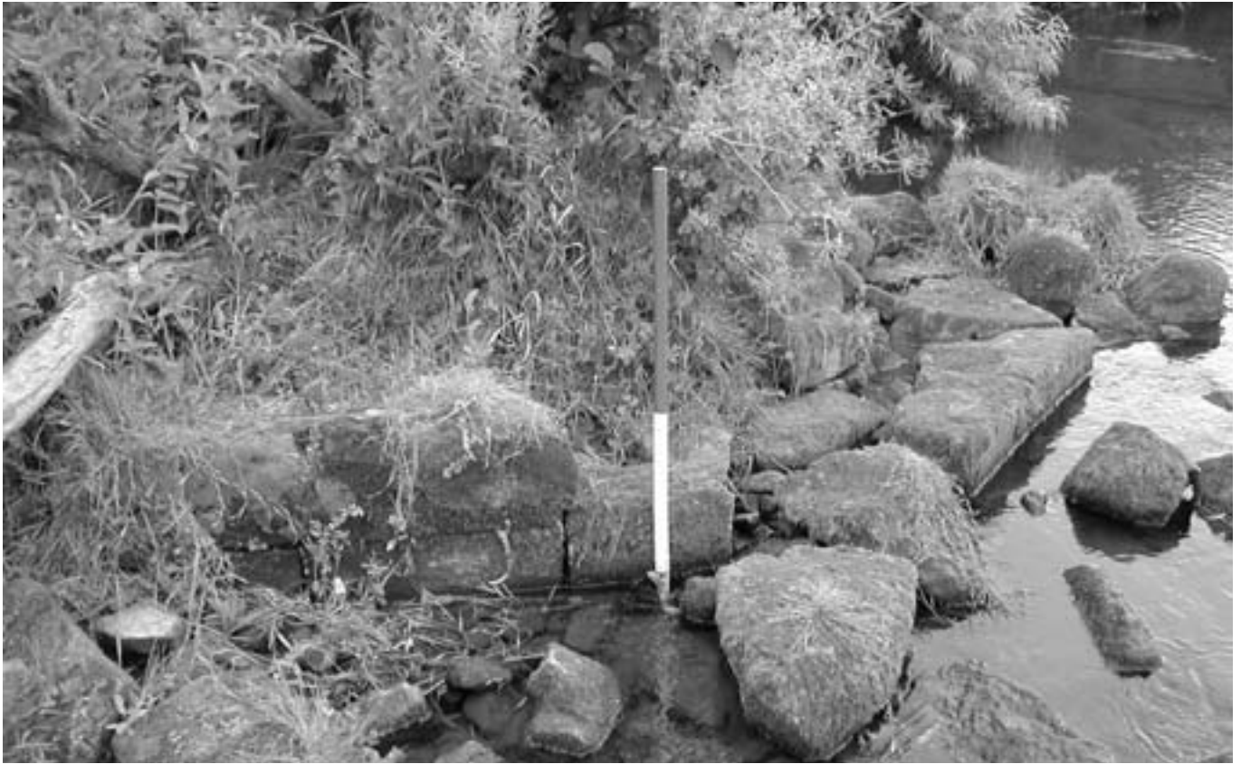
Remains of the east pier of the medieval bridge visible in the River Till.
