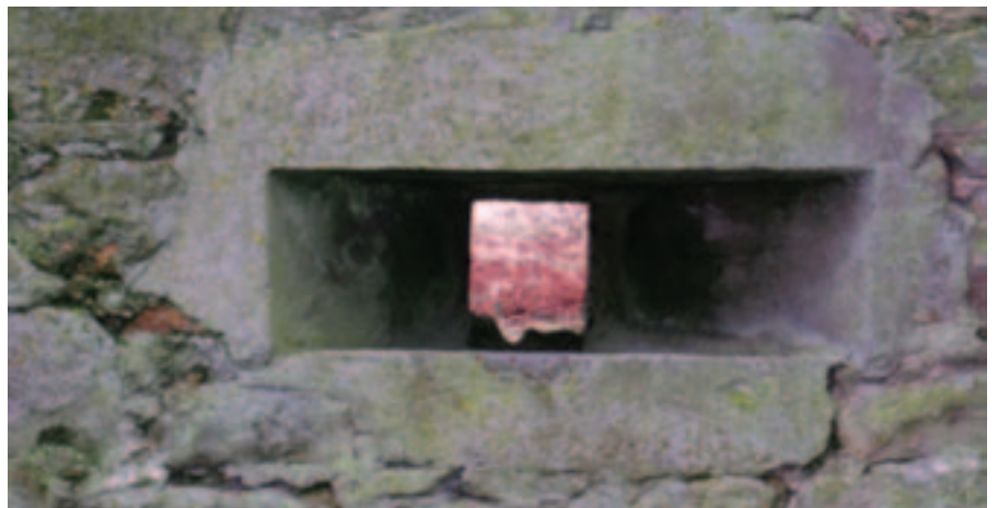
Concrete gun loop inserted between 1939 - 1940.
